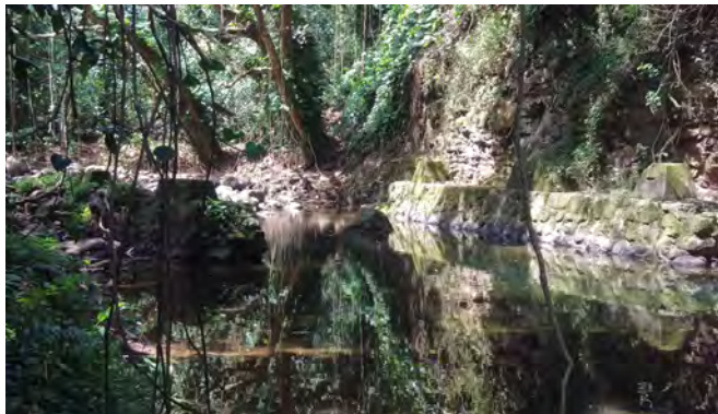
Existing trestle footings
