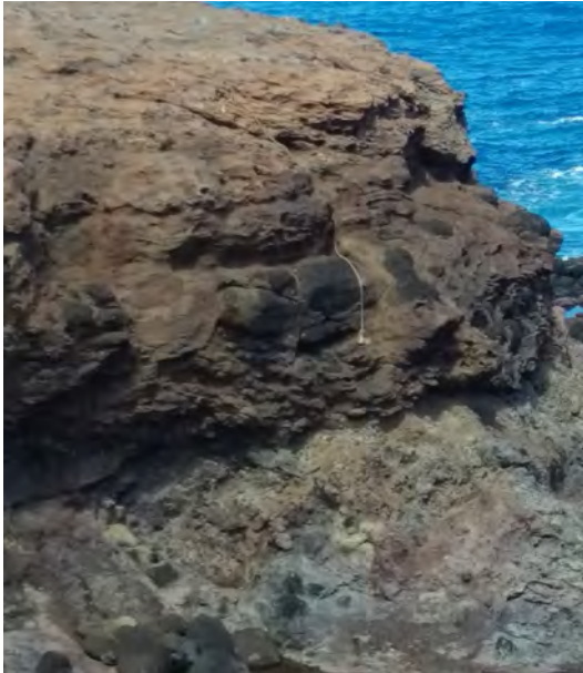
Ropes for access
