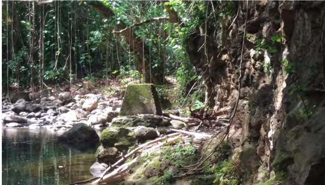
Existing trestle footing
