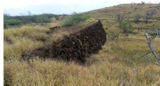
Existing raised railroad bed
